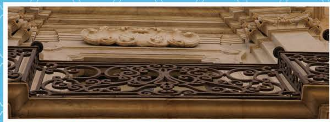
Ingang, Grand Master Palace | MALTA
